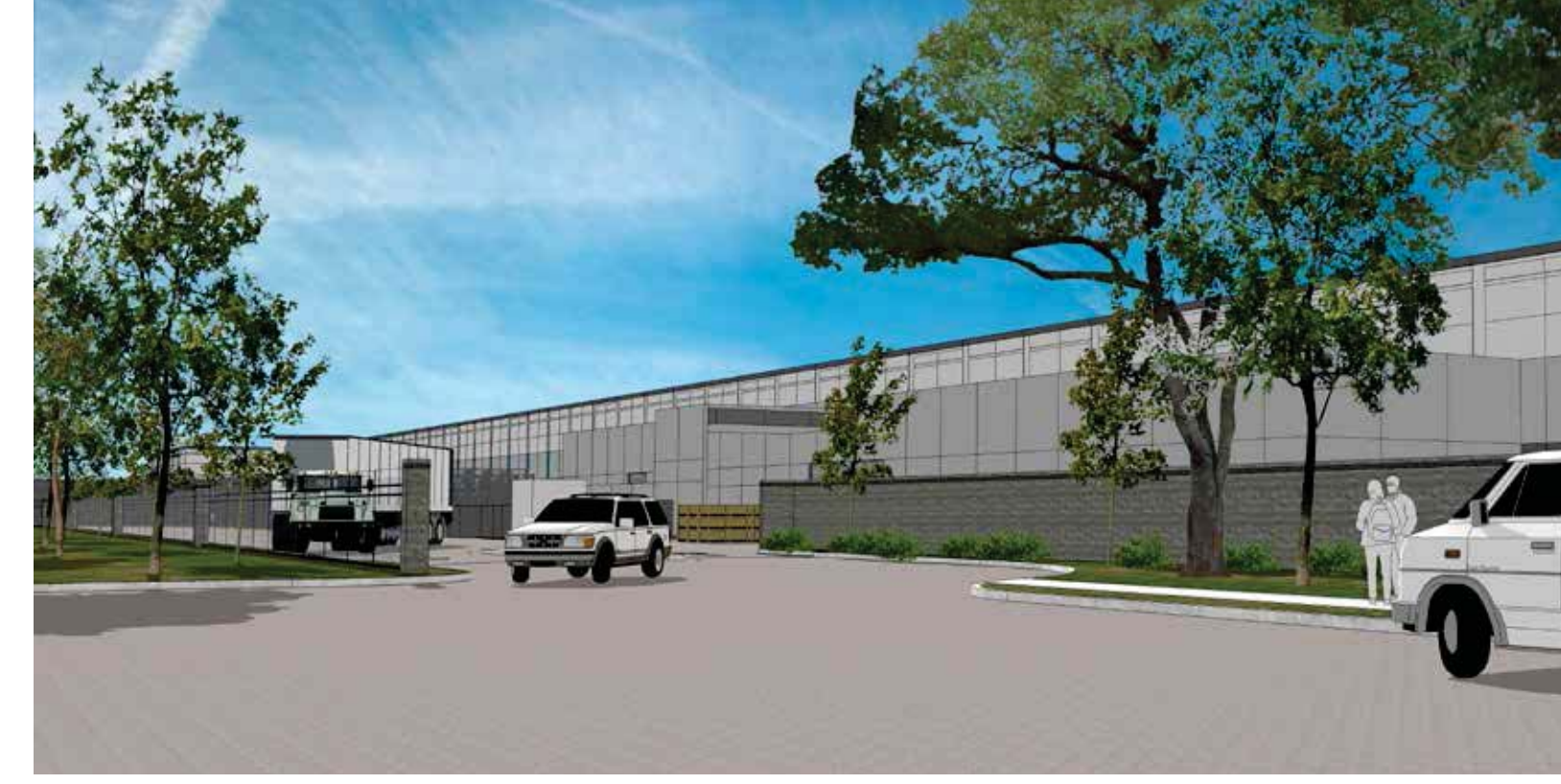
Building 1 Screen Wall - Image 1.3
